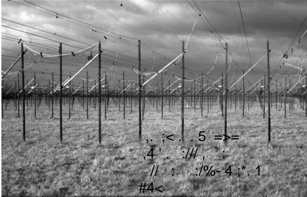
**Figure 4a** The Interplanetary Scintillation (IPS) Array used by Hewish and Bell-Burnell to discover pulsars. The array consists of 1,000 posts hammered into the ground, and strung with almost 200 km of wire, making a total of 2,048 aerials. (Courtesy Graham Woan.)
